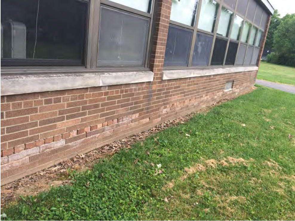
Masonry and mortar deterioration
