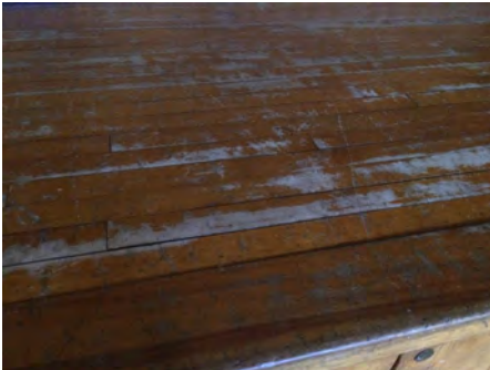
Wood floor in worn condition
