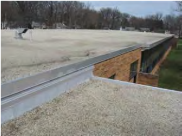
Built-up roofs need replacement
