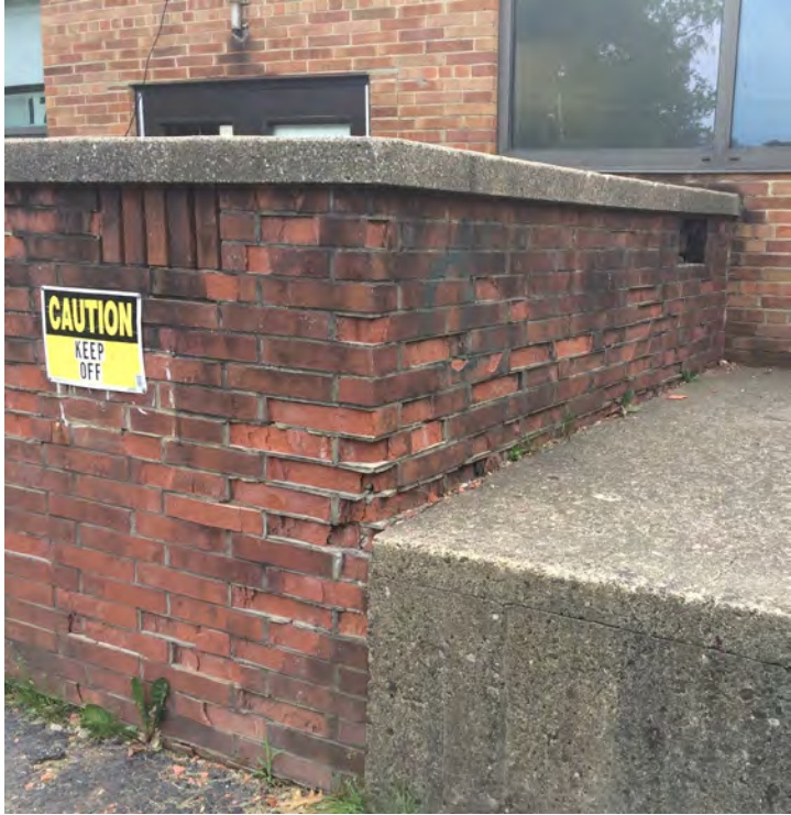
Spalling brick in poor condition
