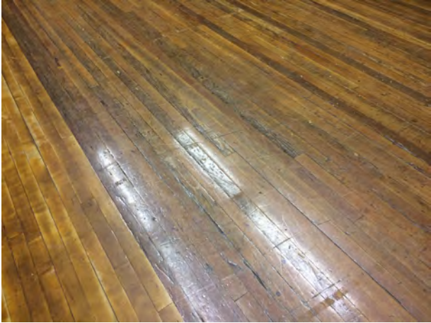
Wood flooring in poor condition
