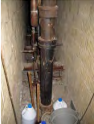
Main sanitary sewer recently had section collapse
